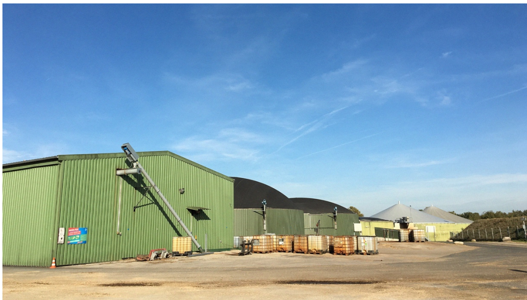
Biogasanlage (Projekt: Next Generation BIOGAS), © Next Generation BIOGAS
